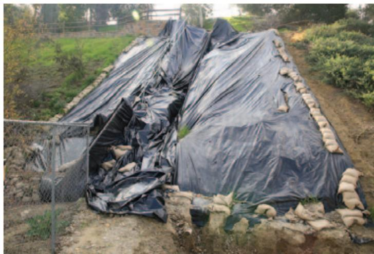
As a temporary control erosion measure, sandbags and plastic sheeting have been in place since January 2017, with City staff monitoring and making adjustments as needed to prevent the damage from expanding.
